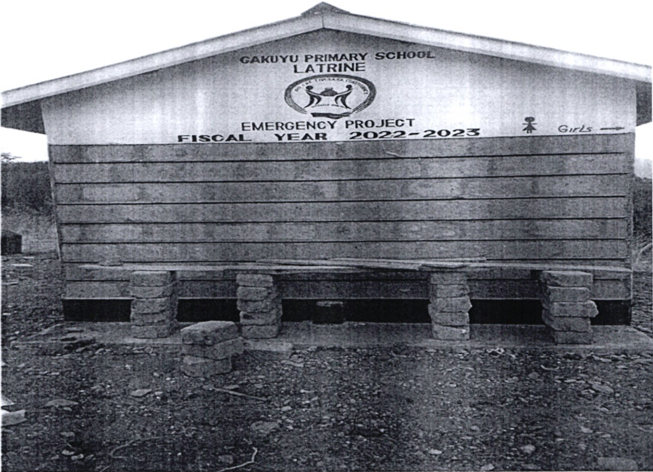
Gakuyu primary school - emergency project
