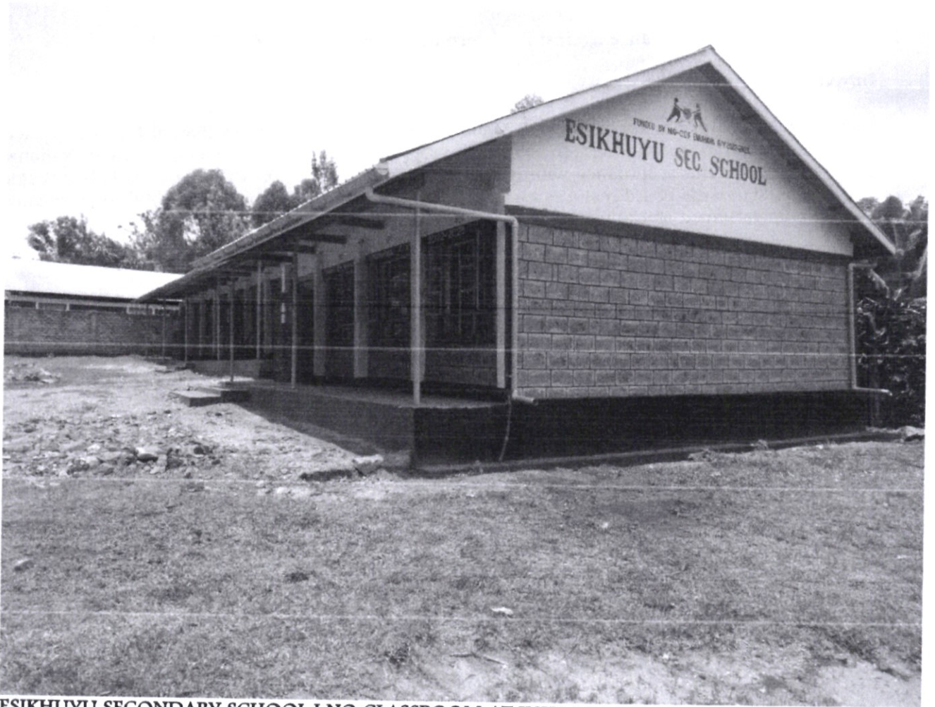
ESIKHUYU SECONDARY SCHOOL I NO CLASSROOM AT KSHS 900,000.00
