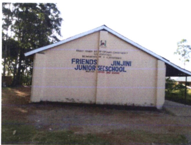
Pic. 3: Jinjini Primary School newly renovated 3No. classrooms fully funded by Hamisi NG-CDF 2022/2023
