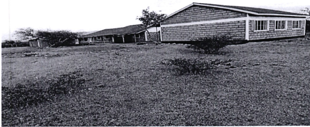
DIMA ADO PRIMARY SCHOOL CONSTRUCTION OF ONE CLASSROOM (approved FY 2021/2022)
