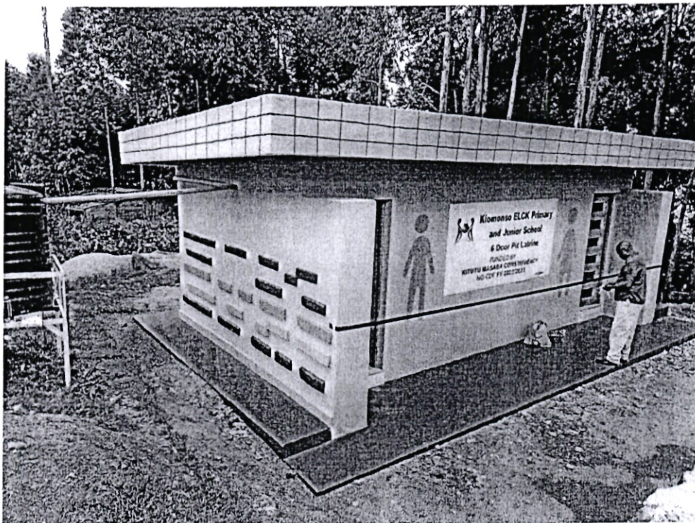
KIOMONSO ELCK PRIMARY SCHOOL TOILET CONSTRUCTION 2022/2023FY @1M
