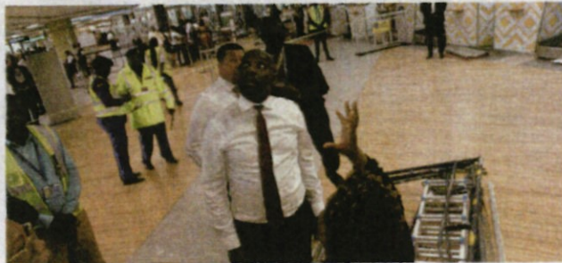
Transport CS Kipchumba Murkomen inspecting part of the roof at the International Departures at JKIA that was under renovation yesterday. [Denish Ochieng, Standard]
