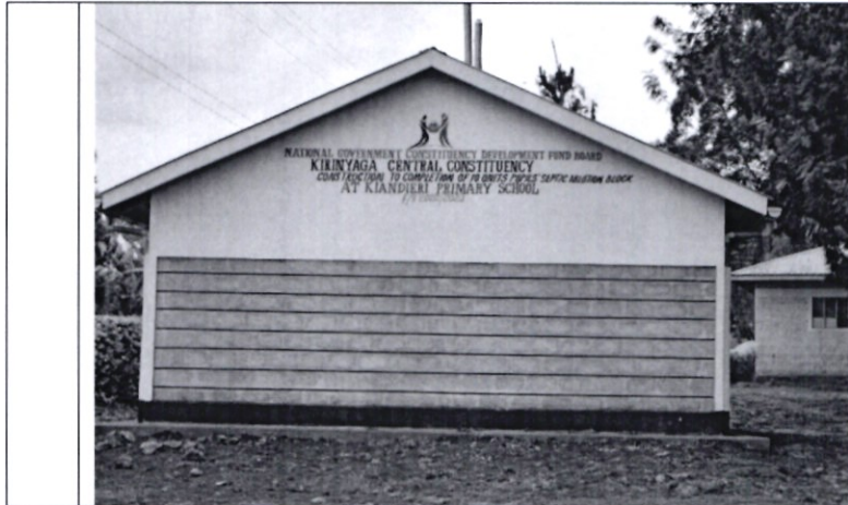
Pupils Ablution Block constructed to completion at Kiandieri Primary school.
