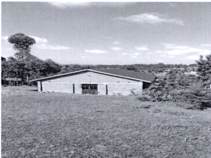
Construction of a dormitory at Biego Secondary school
