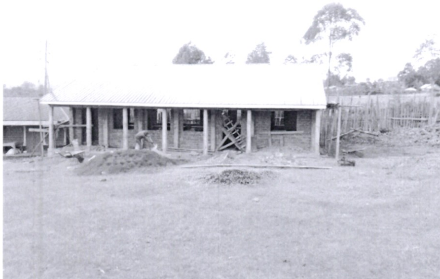
Construction of a Laboratory at St Thomas Moore Riangombe Secondary school
