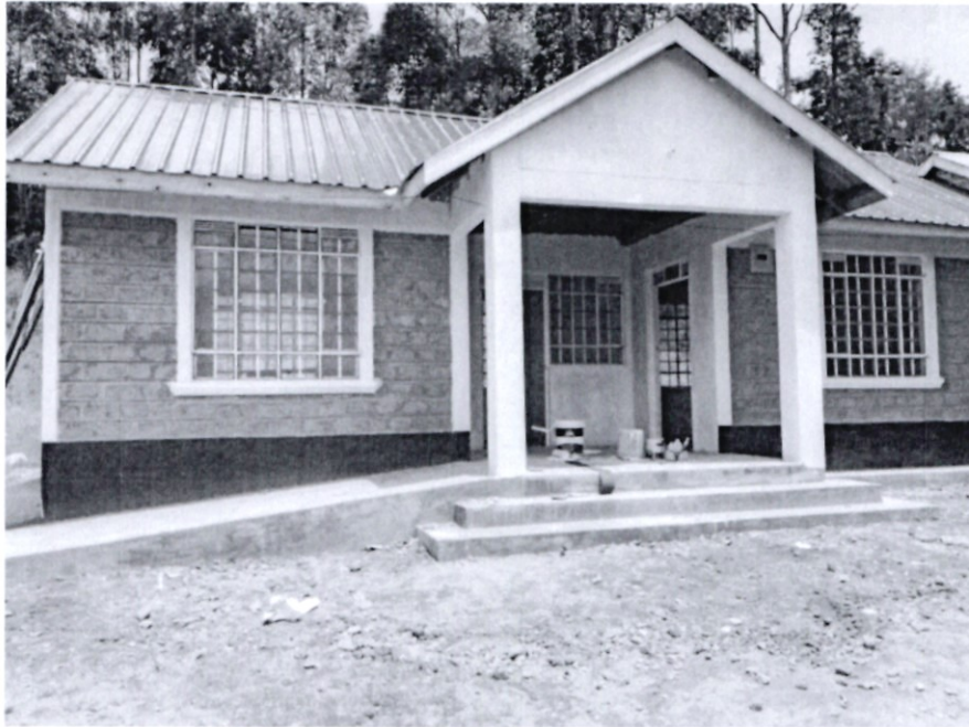
Construction Of Mekenene Chiefs Office
