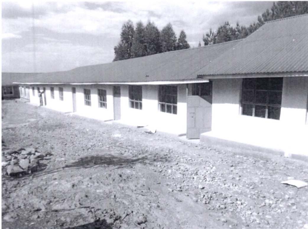
Renovation of seven class rooms at Mogusii Primary school
