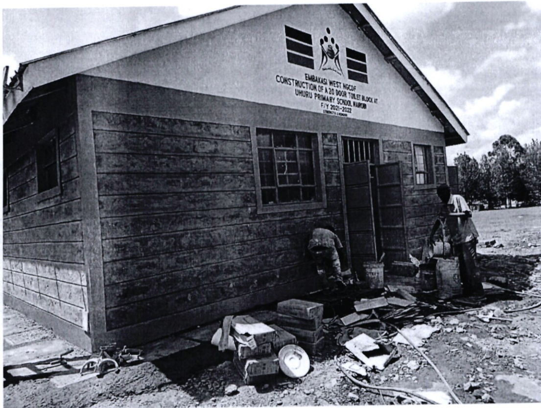
Fig 3:Construction of 20 door ablution block at Uhuru Estate Primary School
