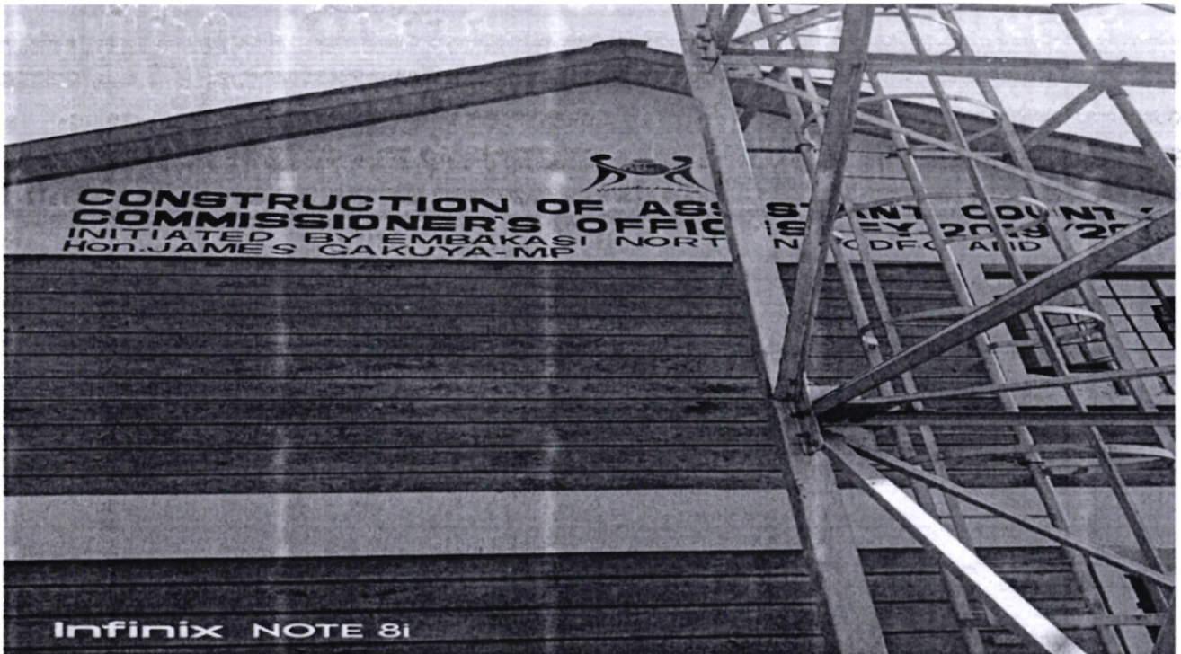
FIG 4: CONSTRUCTION OF DANDORA PHASE 3 ACC OFFICE
