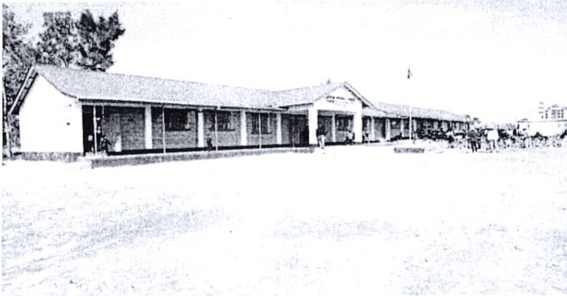
Newly completed Mutuya Primary School which now accommodates over 1000 pupils.
