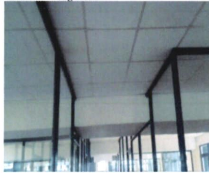
Interior works on the ceiling
