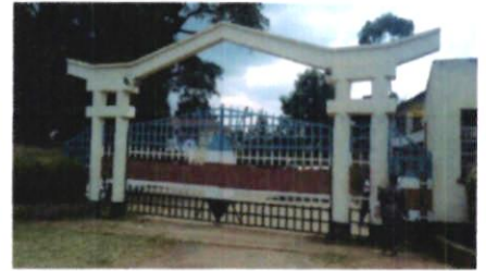
Main Assembly Gate
