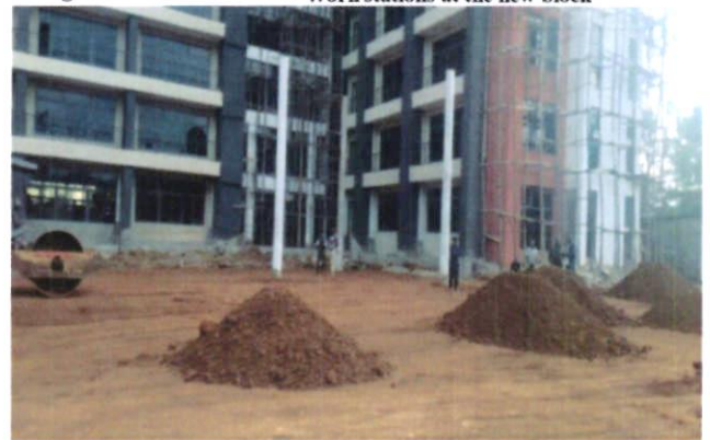
Work in progress- Parking area
