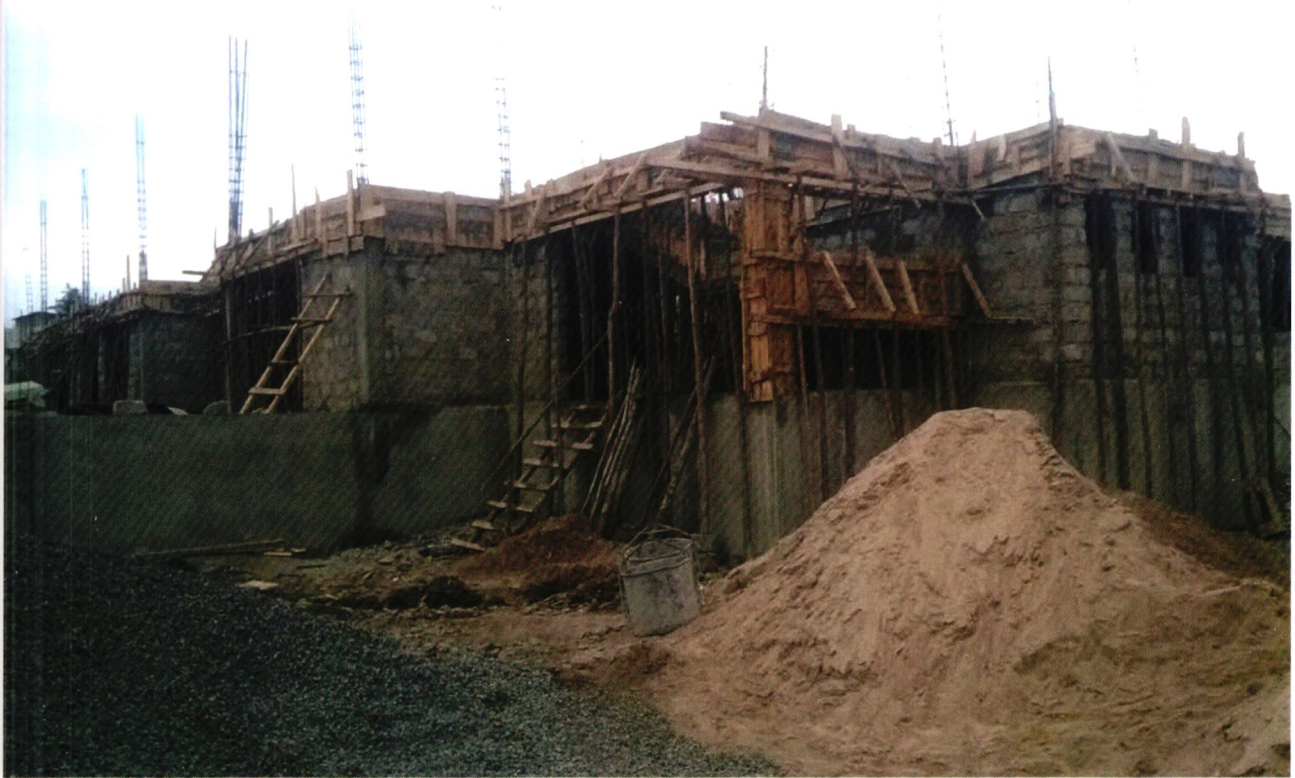
Construction of TSC Office in Bomet County
