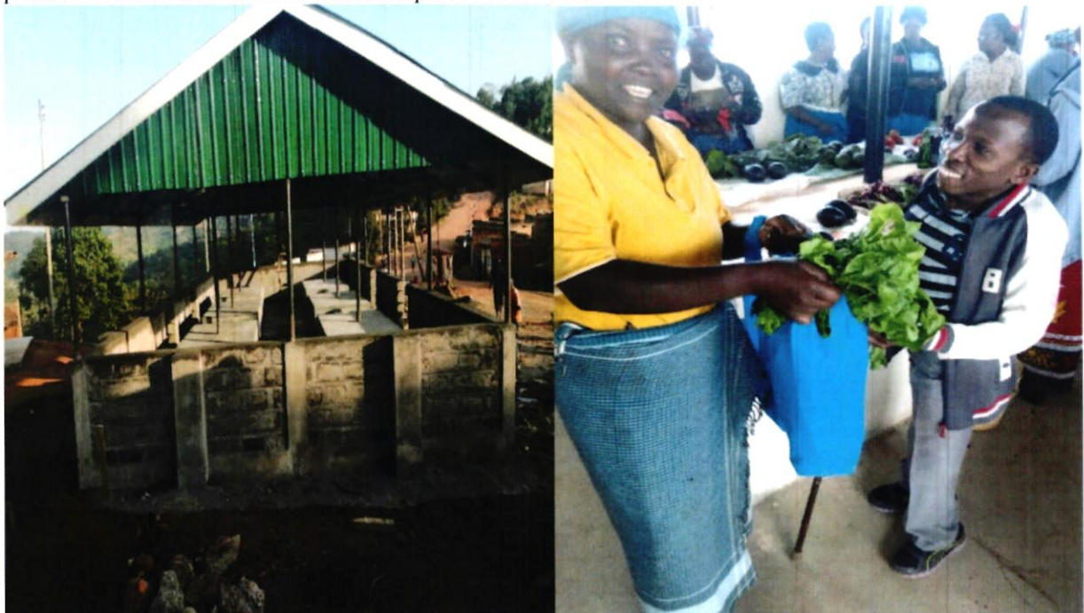
Ikalyoni Market Shed under construction in Kee Ward
