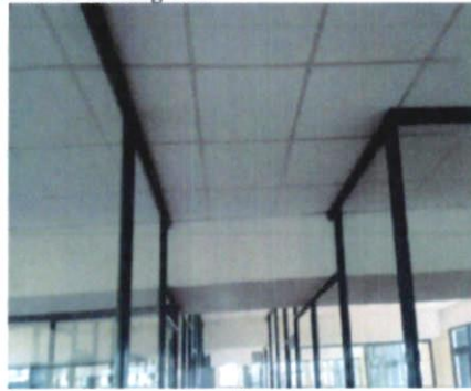
Interior works on the ceiling
