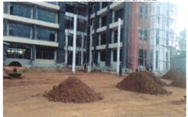
Work in progress- Parking area
