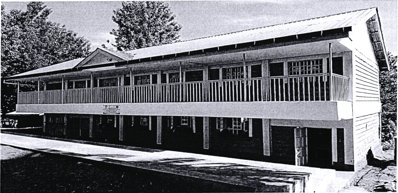
Kiuu Primary School- 2 Classes/Administration Block
