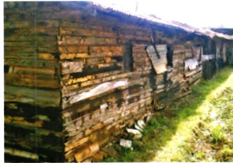
Police accommodation at Kerugoya Police station
