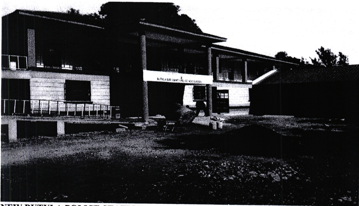
NEW BUTULA POLICE STATION (SECURITY PROJECT)
