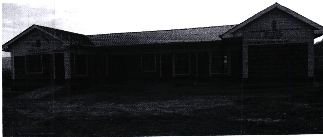
Fig.1.1: Tawa Police Station. Construction of Police Station
