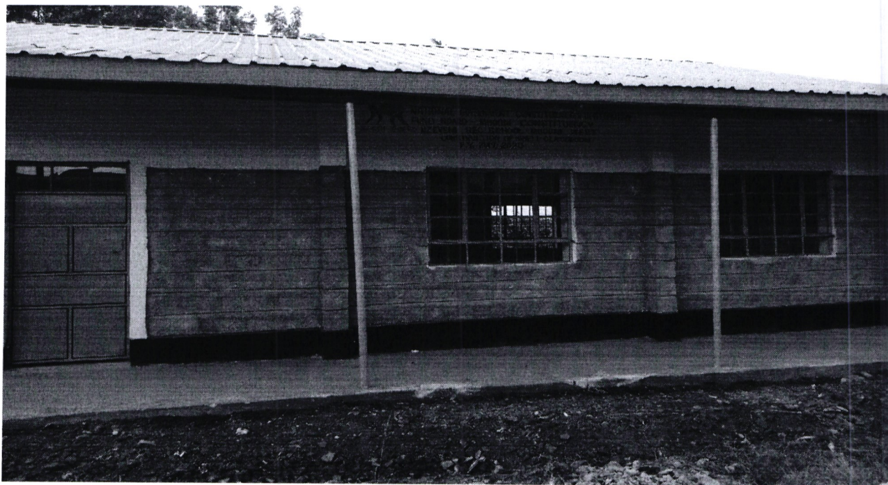
Fig.1.2: Nzeveni Secondary School. Construction of 1 Classroom
