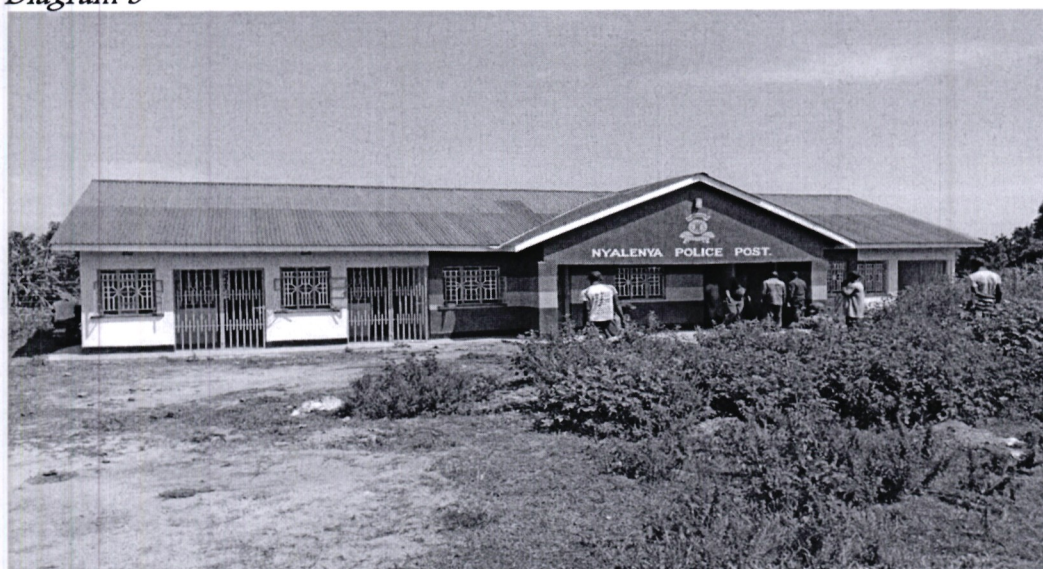
Nyalenya Police Post- construction of police post
