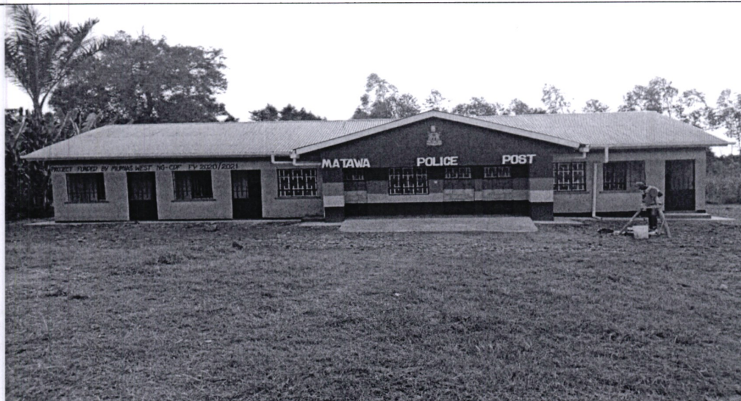
Matawa(Khungema) Police Post - construction of police station
