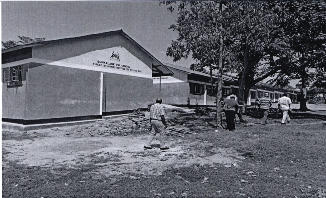
Eshikalame Primary school- construction of 6 classrooms
