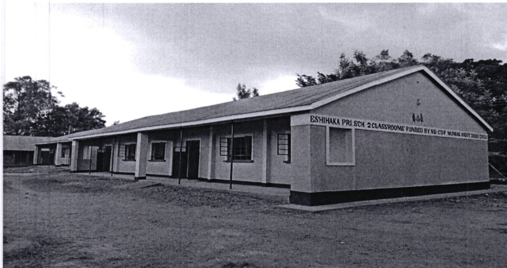
Eshihaka Primary school- construction of 2 classrooms
