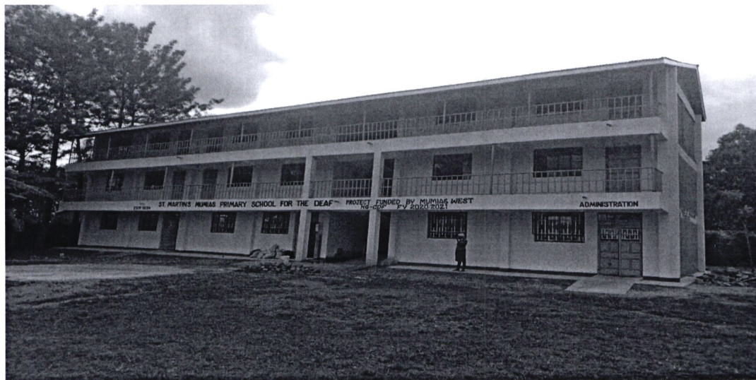
St. Martin School for the Deaf- construction of 6 classrooms and Administration Block
