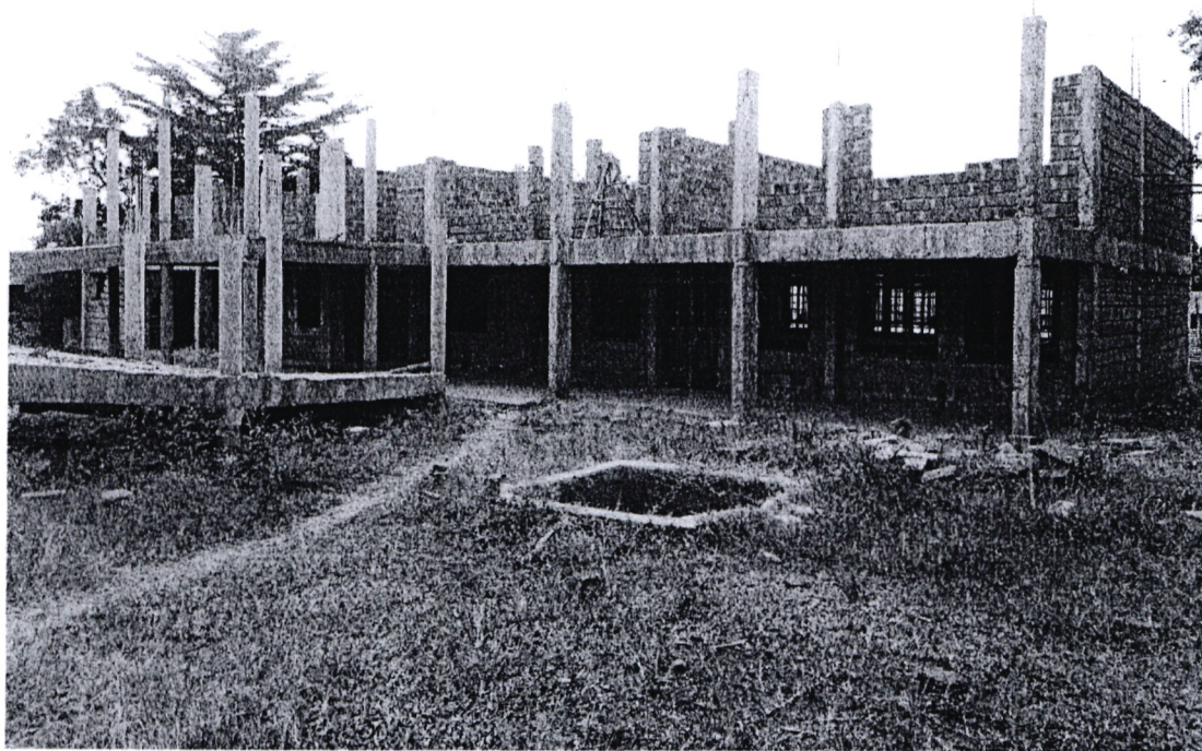
Figure 3 Ongoing tuition and administration block at Busia Township Primary School
