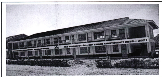
Wamalwa Kijana Memorial High School Storied Building with six classrooms
