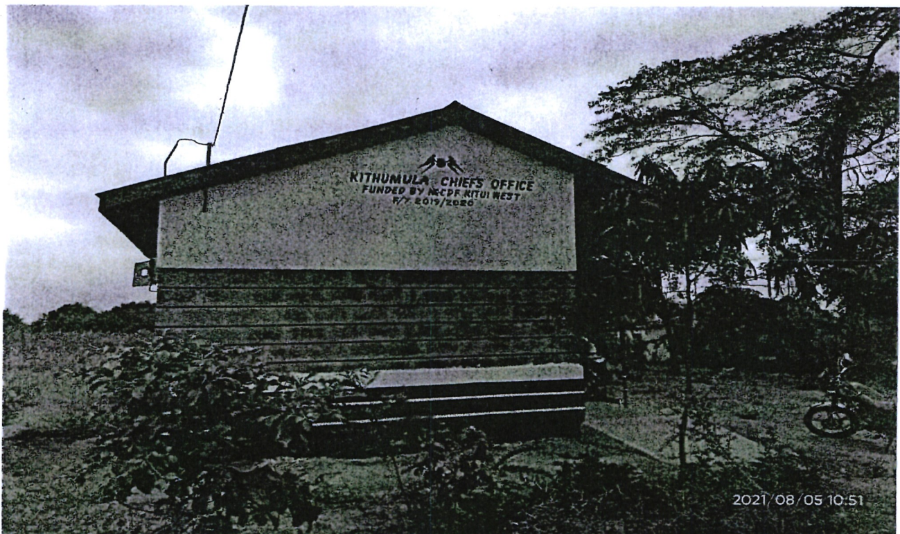
Figure 3: Construction of Kithumula Chief's office
