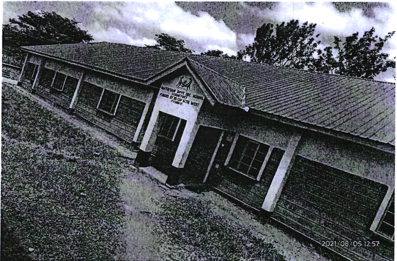
Figure 5: Construction of a dormitory at Matinyani Boys Secondary School
