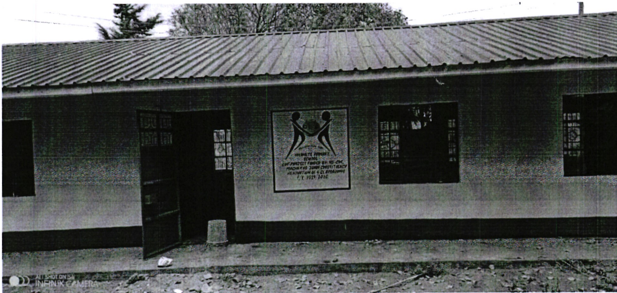
Yakamete Primary School – Renovation of 3 classrooms
