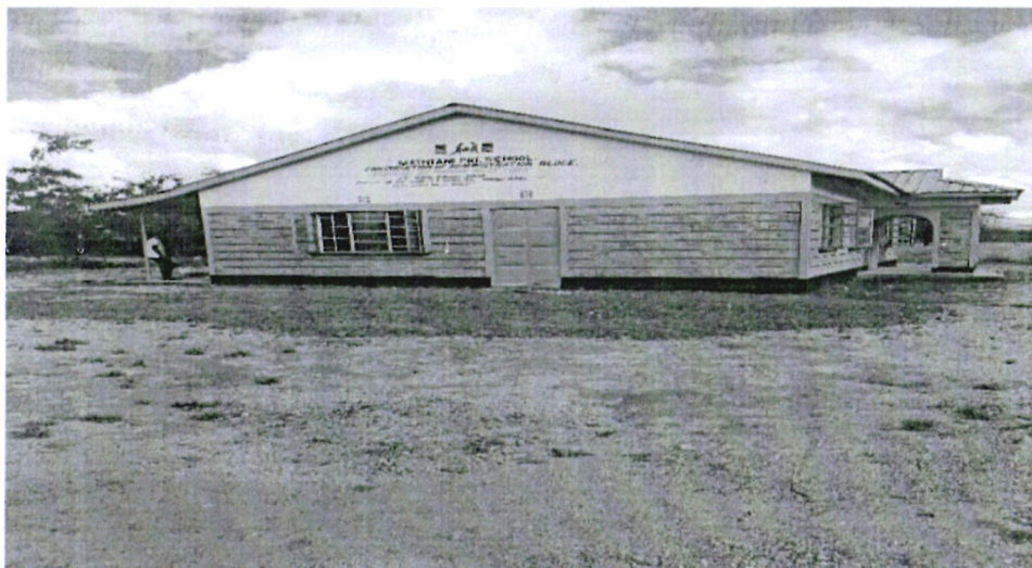
FIG 1.2: Administration block constructed at Mathiani Primary School, completed FY 2020/2021 to improve teachers working environment.
