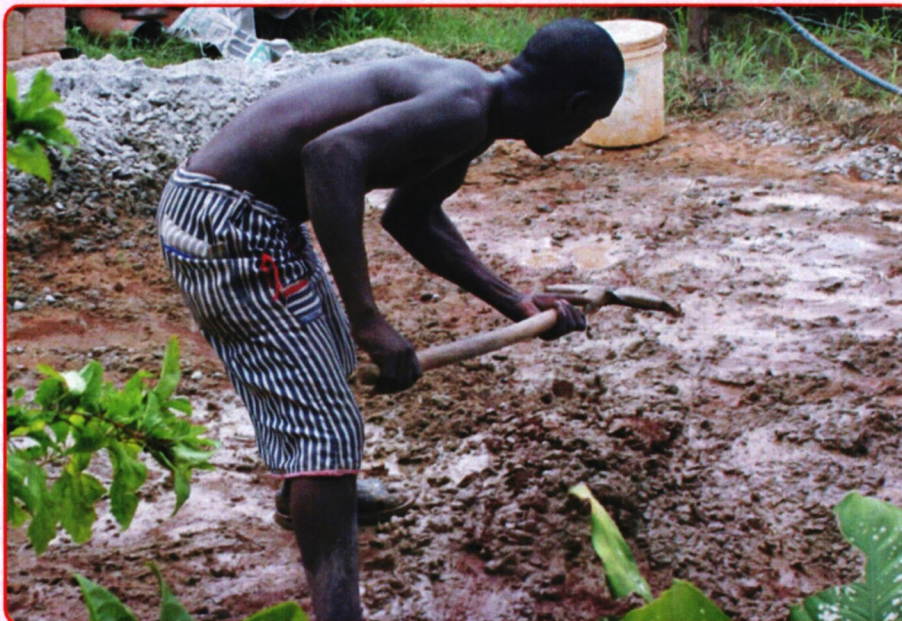
A skilled masonry inmate at work at Malindi Prison
