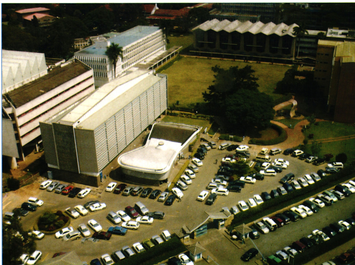
Aerial View of the Main Campus.
