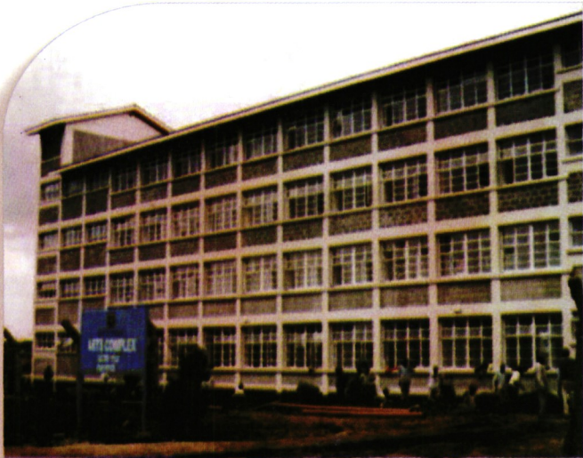
Art Complex phase 2 under construction
