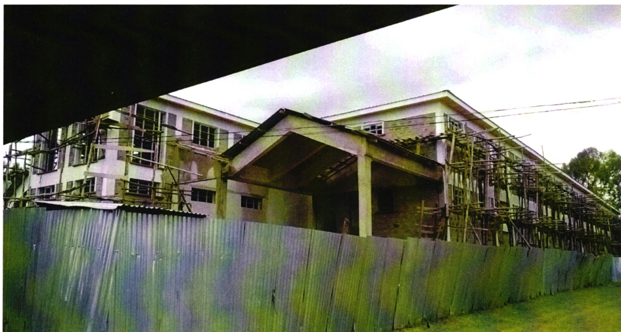
Figure 2 Stalled Trauma Centre within the premises of Nakuru Level 5 Hospital
