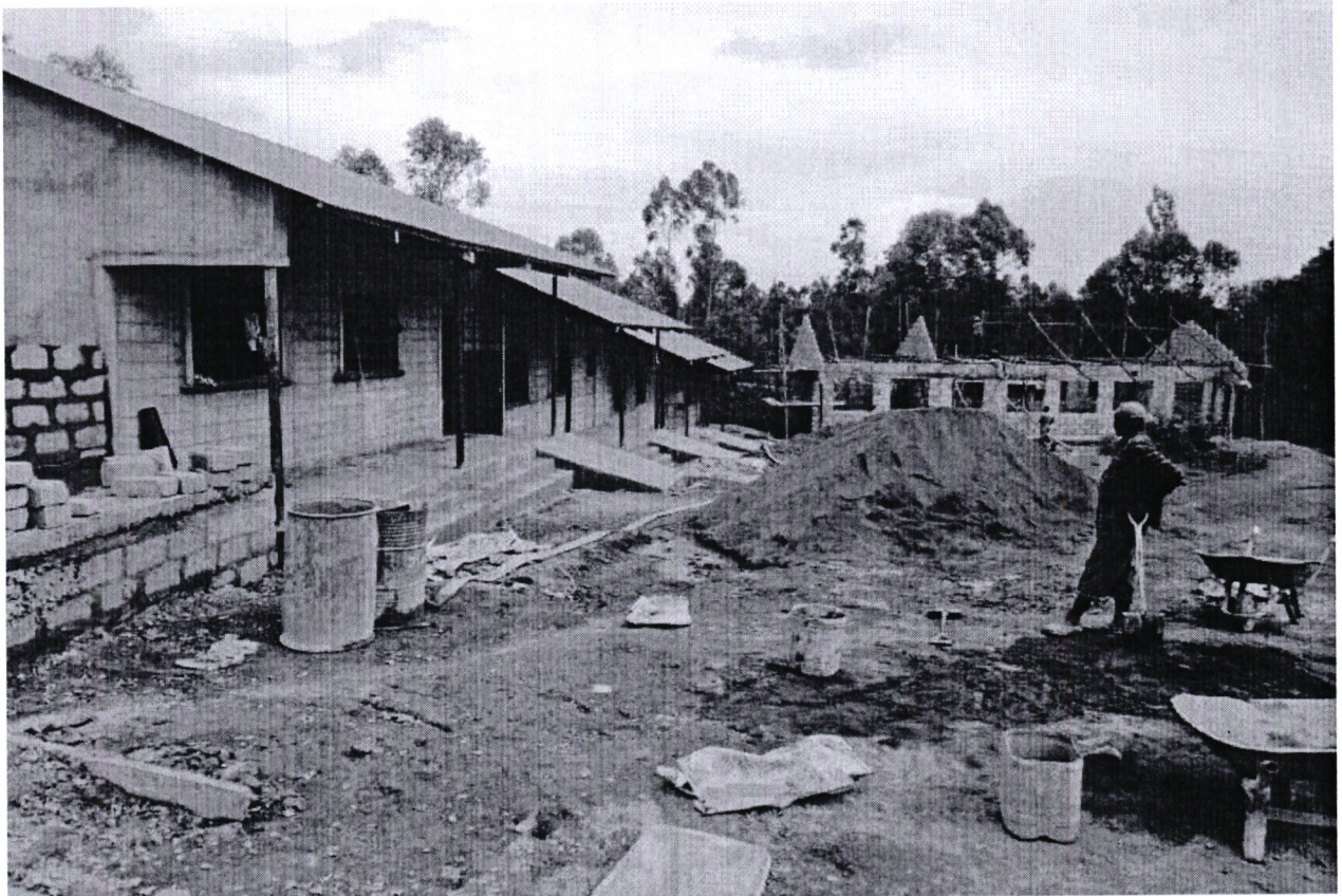
On going construction of 5no classrooms at Esibeye Secondary school
