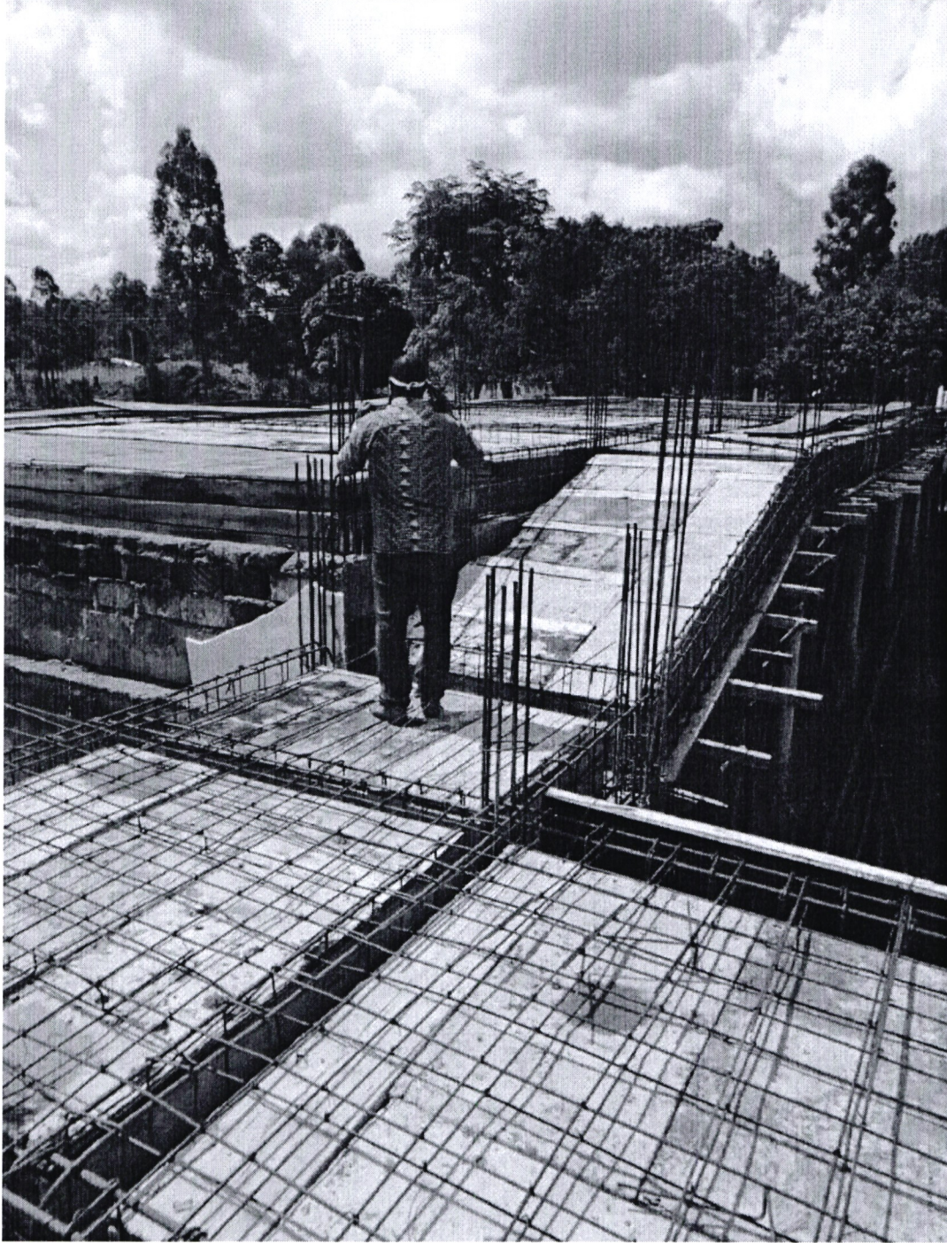
On going construction of 8no classrooms at Esibeye Primary school
