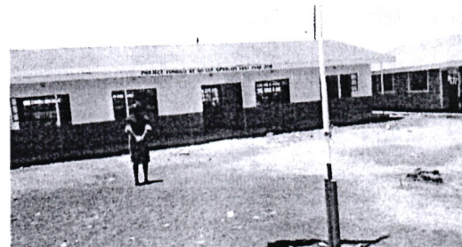
Construction of a classroom at Simboiyon
