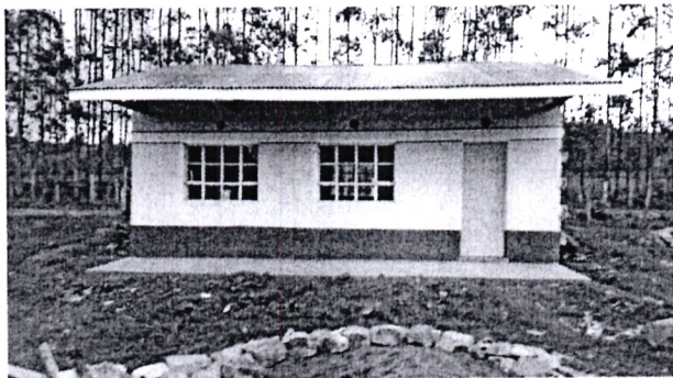
Construction of a classroom at Tiritcha Pry School
