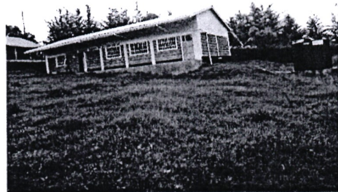
Construction of two Classrooms at Ringa Sec School
