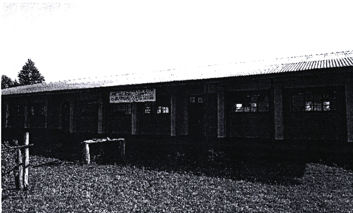
Fig 4: Shows a newly constructed 3 classrooms Block at Lufwindiri primary School Webuye East Constituency for enhancing learning environment.
