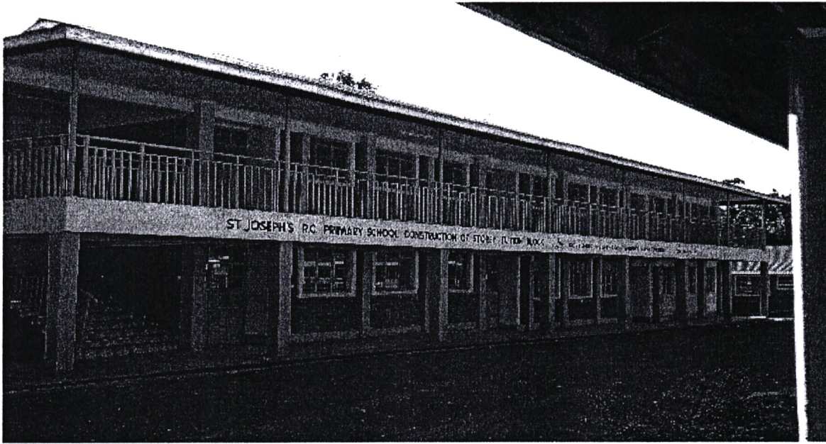
Fig 3: Shows a newly constructed 6 classrooms storey Block at St. Joseph RC Primary School Webuye East Constituency for enhancing learning environment.
