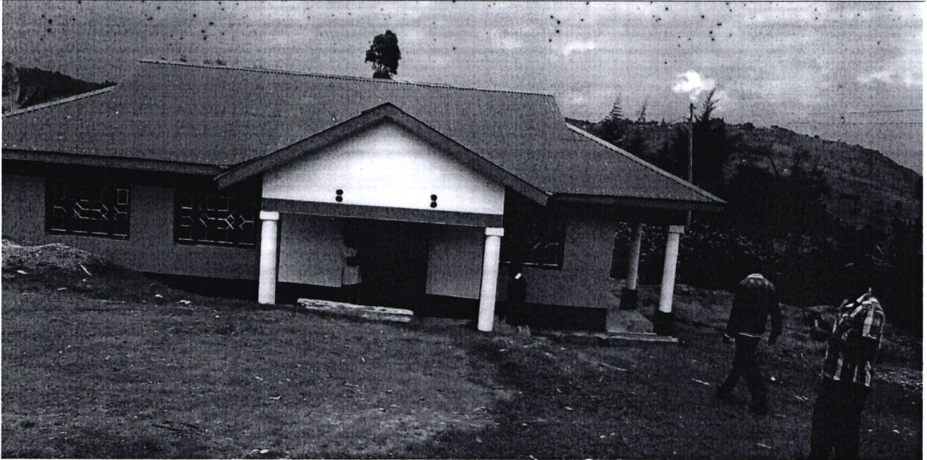
Kapterit Assistant Chief's office- Ongoing construction
