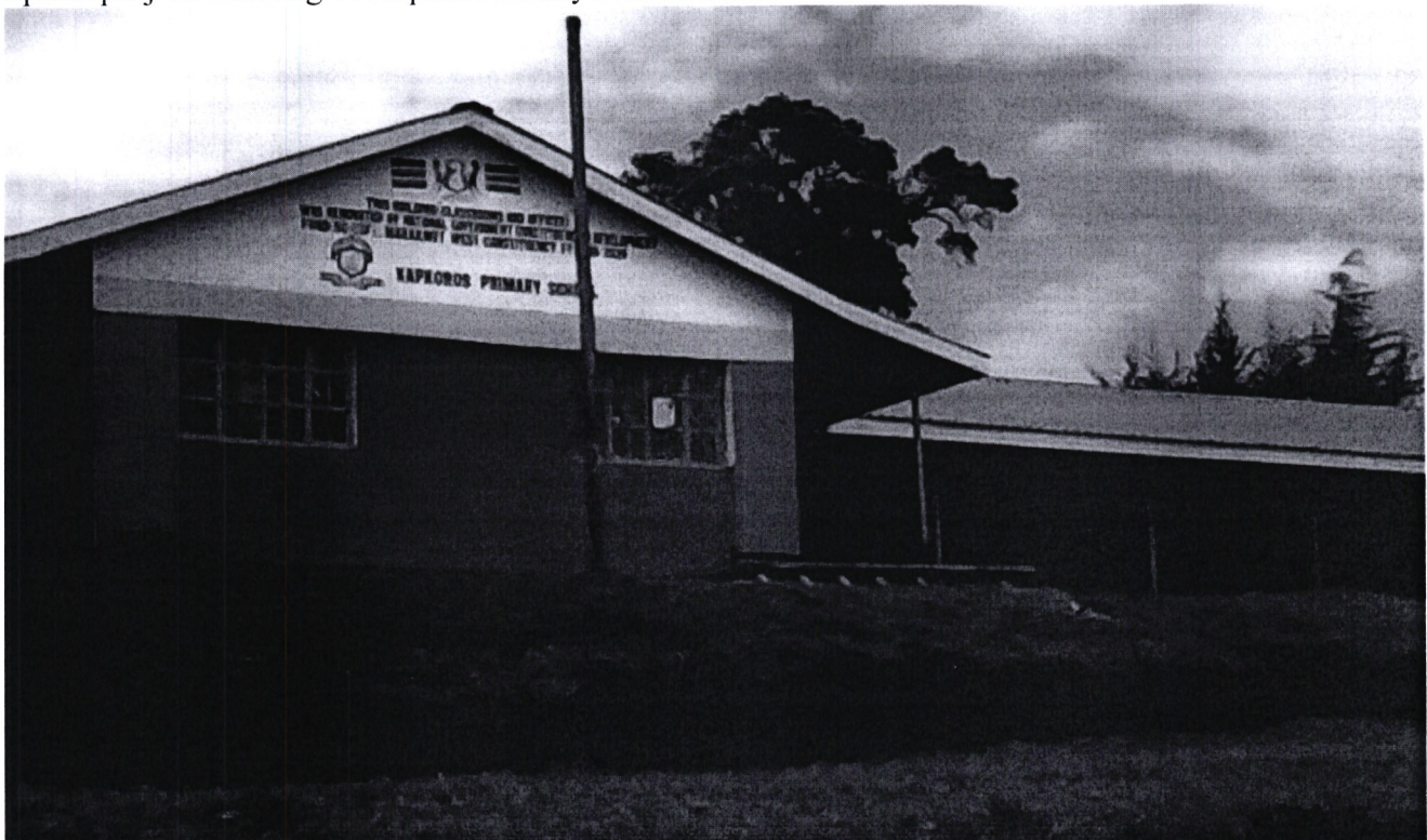
Kapkoros Primary School –Renovation of classrooms
