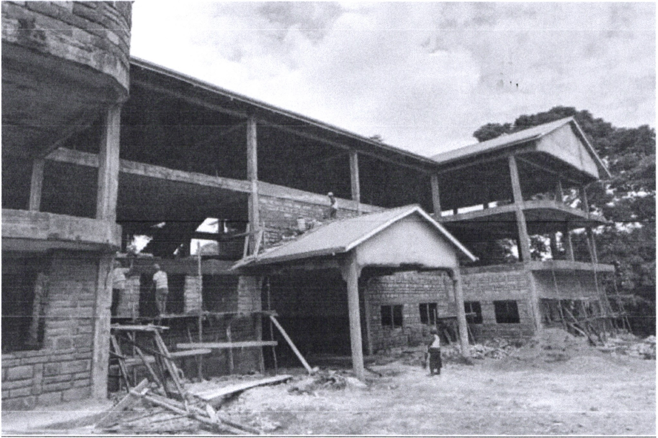
Ongoing construction of NG-CDF Office Block
