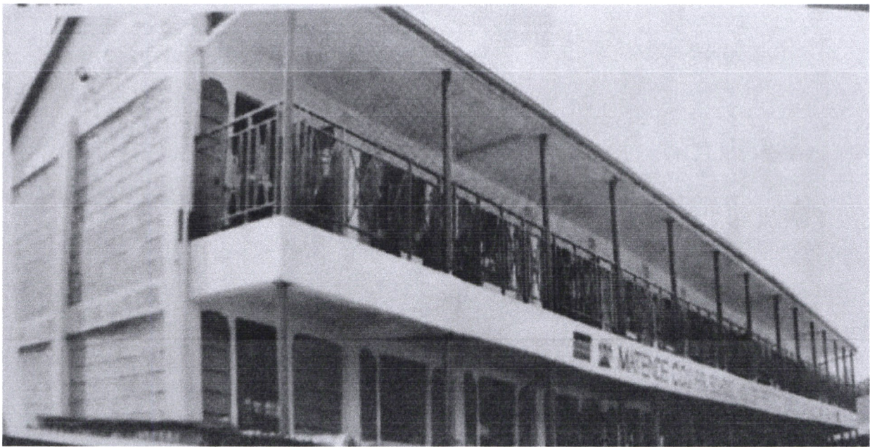
Matende Primary School –Construction of 8 No Classrooms Storey
