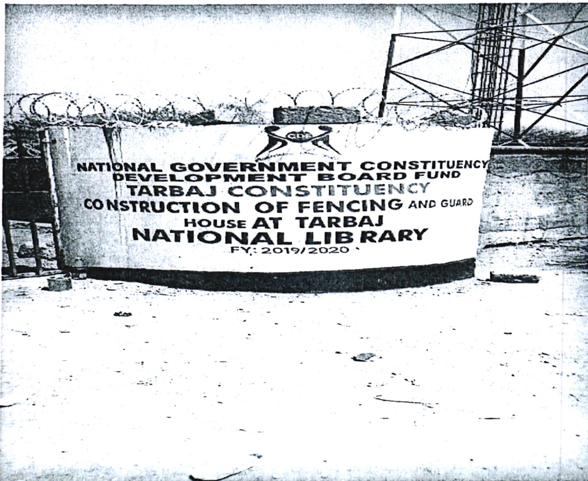
Free tion of chainlink fence with concrete posts 350m *350m , barbed wire , with gate and guard house for ksh 3,500,000/= at Tarbaj sub-county National library.
