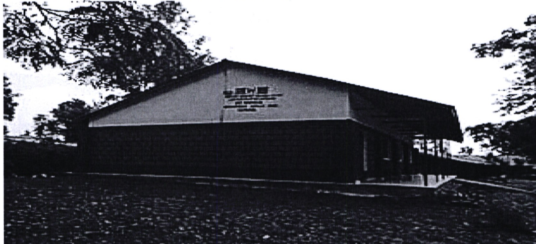
BUKOKHOLO GIRLS SEC. SCHOOL – CONSTRUCTION OF ONE CLASSROOM
