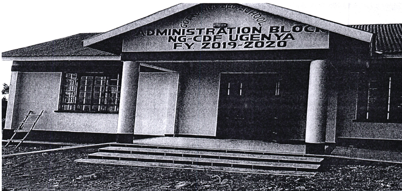
Got Nanga Secondary School – Administration Block
