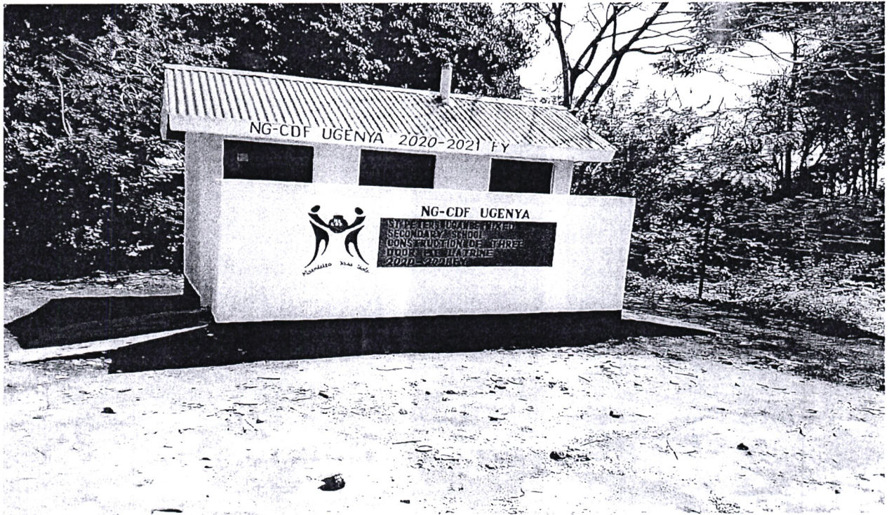
Ugamba Secondary School – Construction of Three (3) Classrooms and a Three (3) Door Latrine
