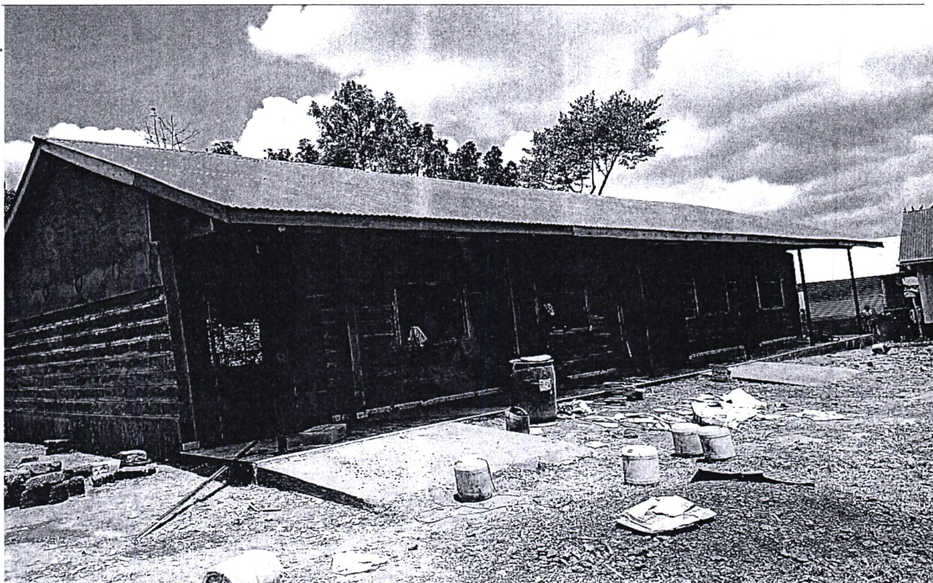
Bar Odar Secondary School – Construction of Two (2) Classrooms.
